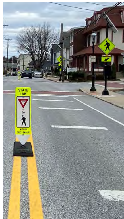
Rectangular Rapid Flashing Beacon (RRFB) and In-Street Pedestrian Crosswalk Sign in Malvern, PA
