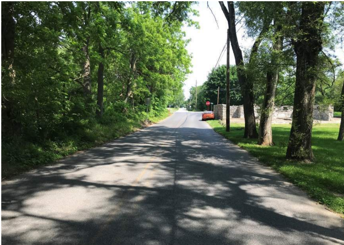
Direction / Road: NB S Ridge Road Approach / Departure: Approaching York Road (SR 0074) Distance: 200 Feet
