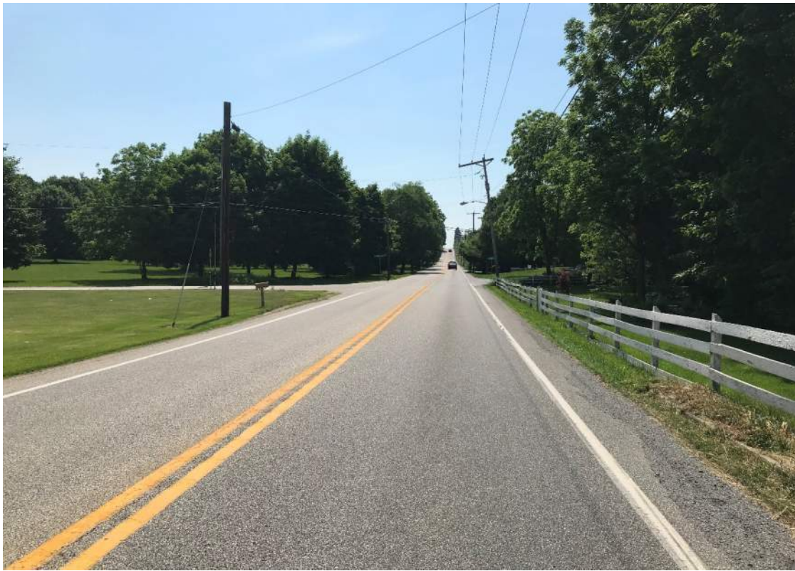
Direction / Road: EB York Road (SR 0074) Approach / Departure: Approaching S Ridge Road & S Middlesex Road Distance: 200 Feet
