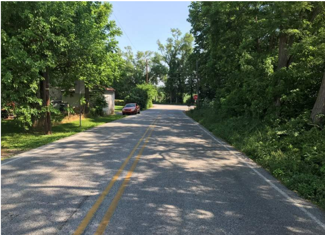
Direction / Road: NB E Springville Road Approach / Departure: Approaching York Road (SR 0074) Distance: 200 Feet
