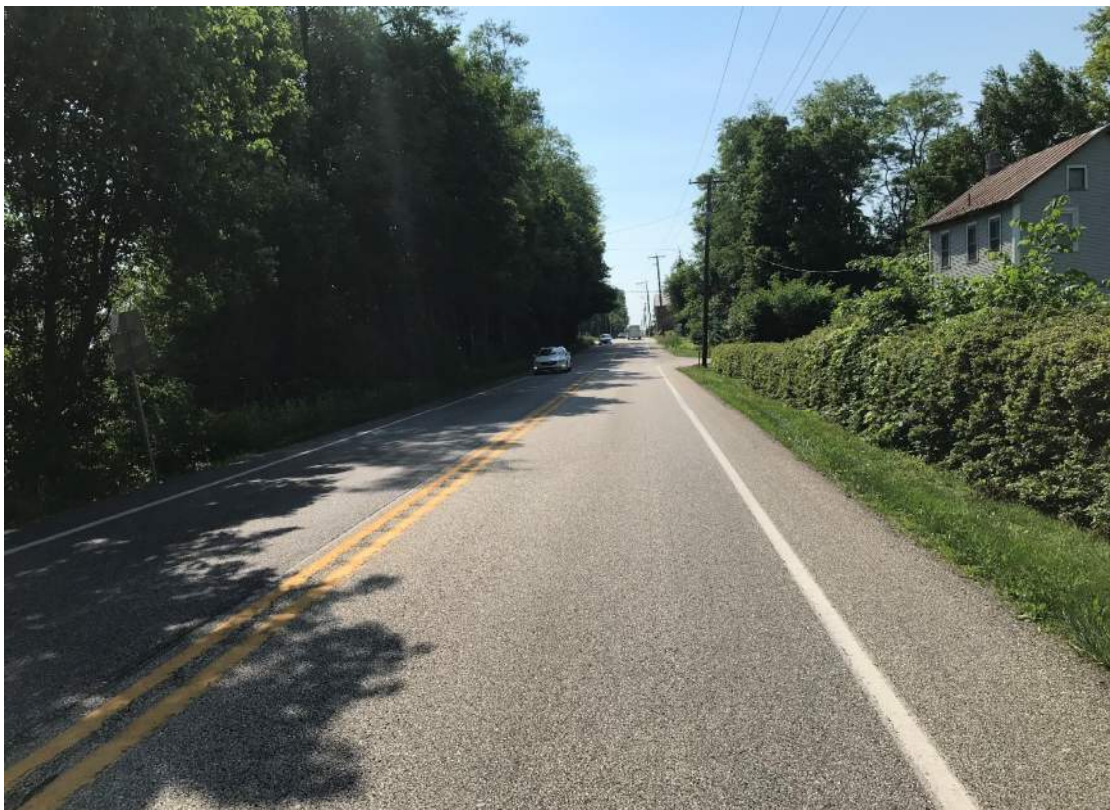
Direction / Road: EB York Road (SR 0074) Approach / Departure: Approaching E Springville Road Distance: 200 Feet
