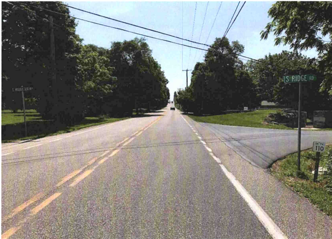
Direction / Road: EB York Road (SR 0074) Approach / Departure: Approaching S Ridge Road & S Middlesex Road Distance: 50 feet
