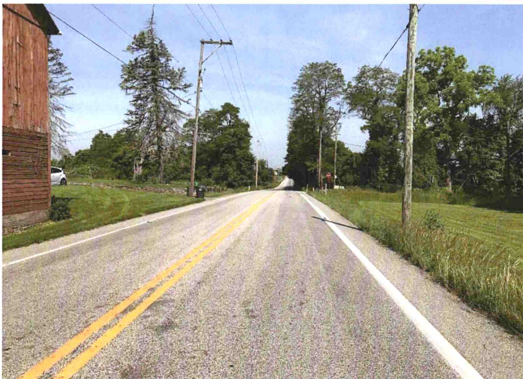
Direction / Road: WB York Road (SR 0074) Approach / Departure: Approaching Shughart Road Distance: 200 Feet
