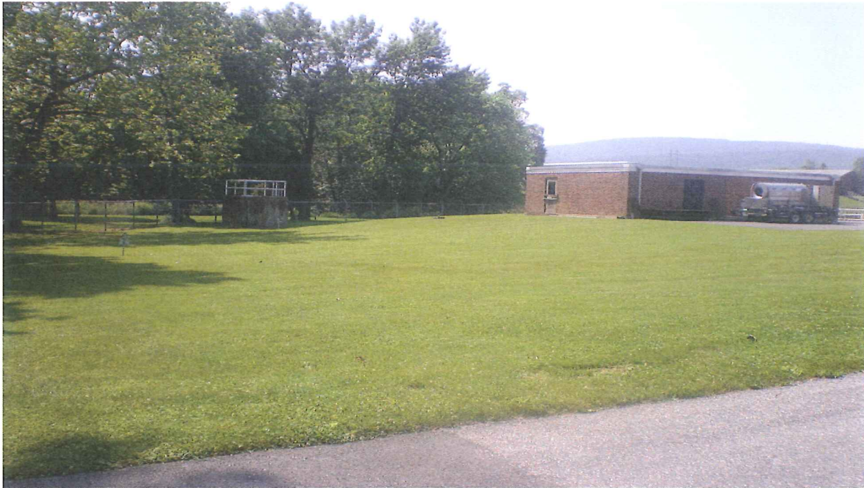
The area between the existing filter building (bottom picture on the right) and the fence on the northern side of the plant is the proposed site for the construction of the clarifiers. The existing filter building is proposed to be converted into tertiary filter system or UV disinfection system.
